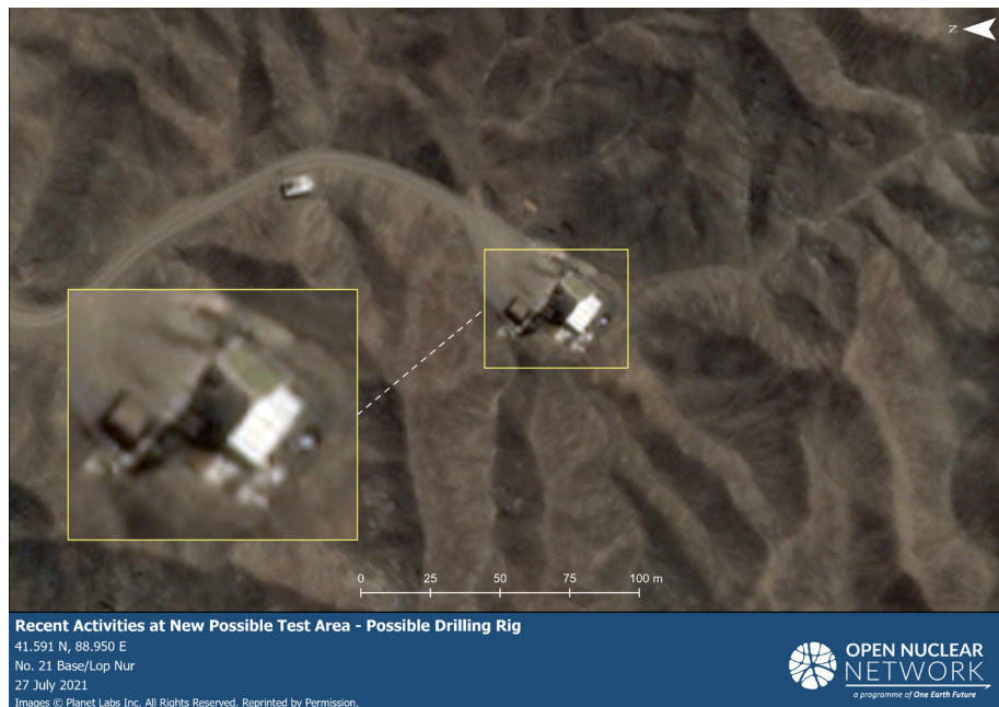
Figure LN-6: A possible drilling rig was installed in Area 4 of the new possible test area (Image 12) as early as 27 July 2021 and seemed to have been dismantled by September 2021.
