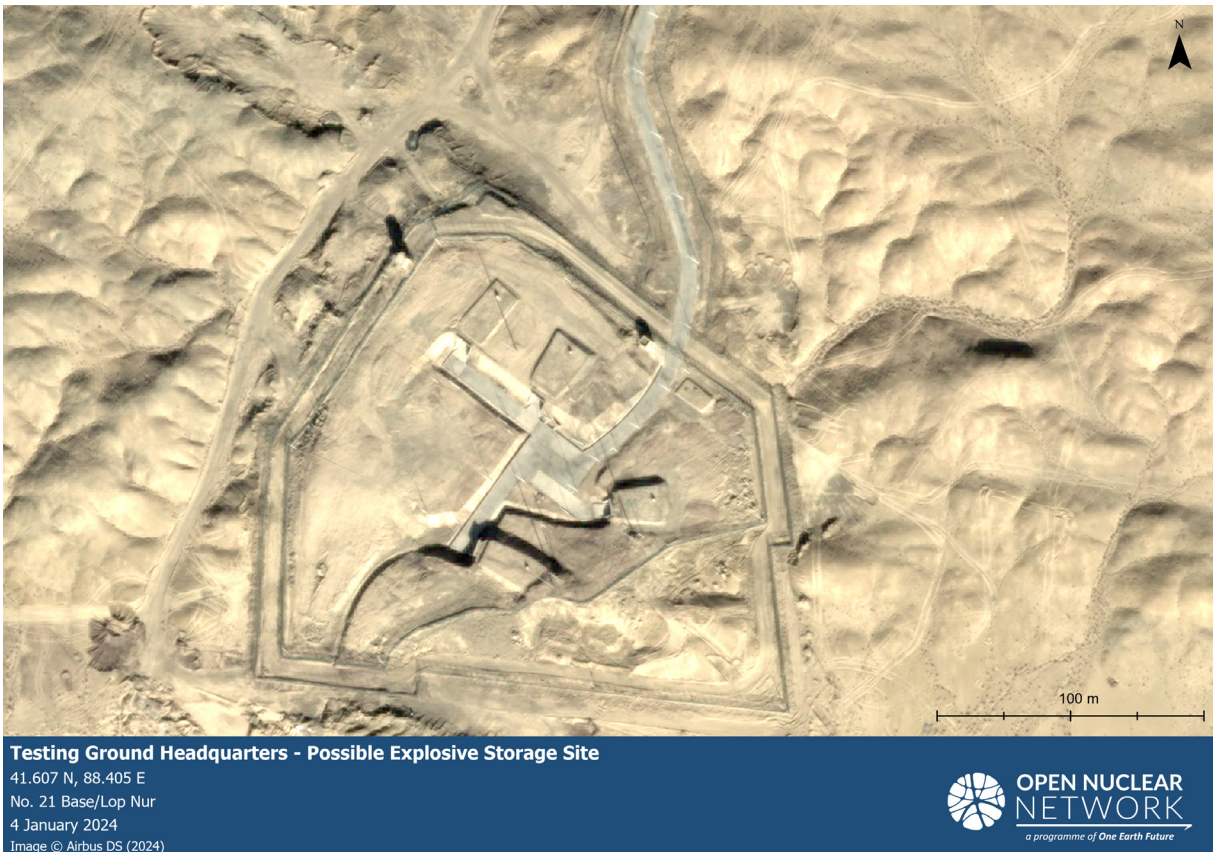
Figure LN-3: Another possible explosive storage site (construction started in 2021). Multiple lightning arresters, berms, bunkers, and double-layer fencing suggest that this site may be associated with the handling of explosives.
