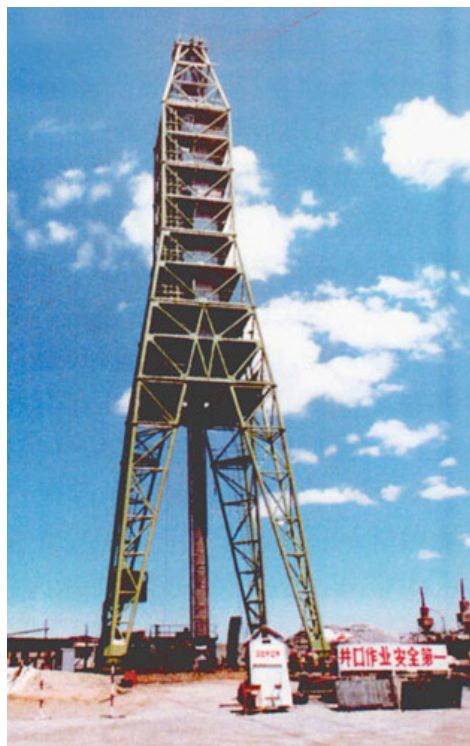
Figure LN-5: A drilling rig used to construct a vertical shaft for a Chinese underground nuclear test. Image: 81.cn 90
