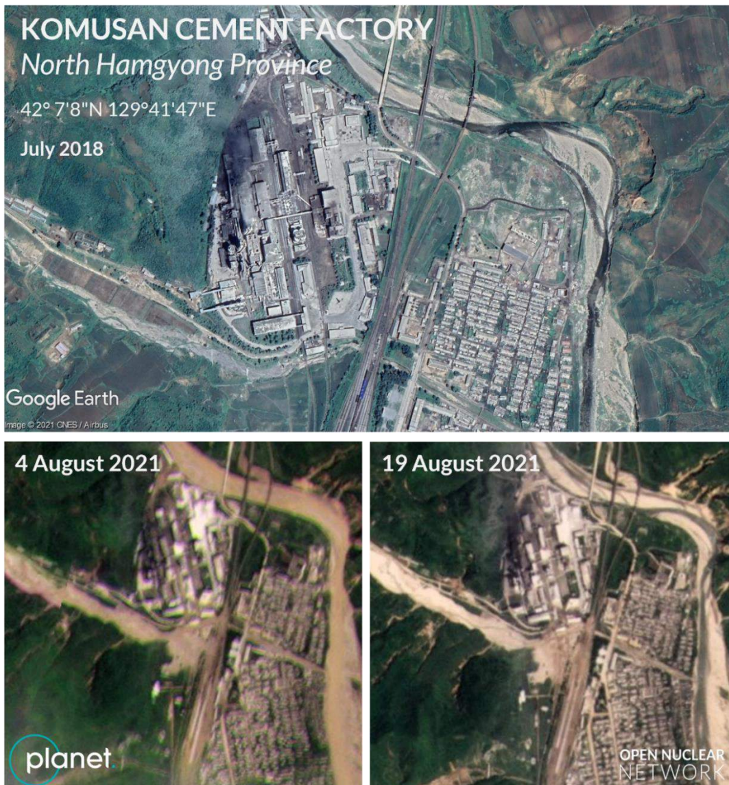
Figure 18. Satellite imagery showing flooded railways near the Komusan Cement Factory (bottom left). Traces of the damage to railways can be observed in satellite imagery from 19 August (bottom right). Images: Google Earth and Planet Labs Image © 2021 Planet Labs Inc. All Rights Reserved. Reprinted by permission
