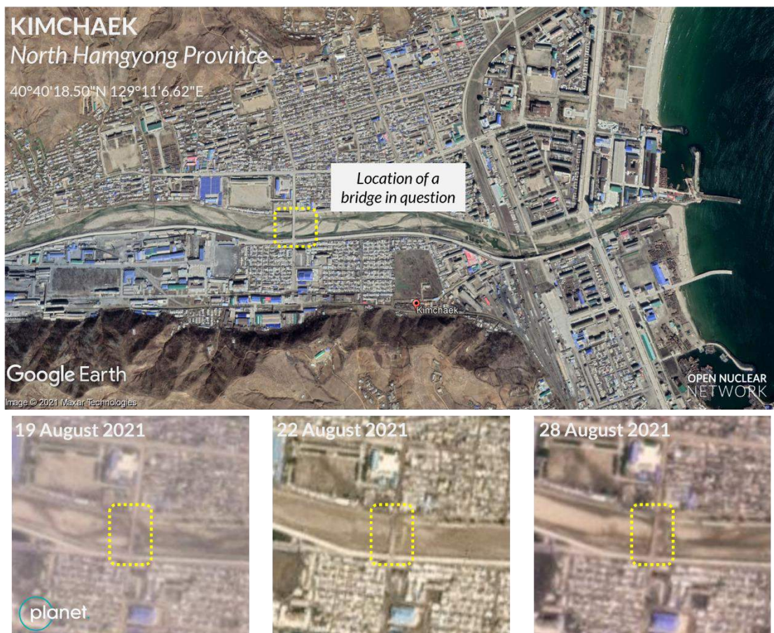
Figure 23. Overview of Kimchaek and the location of a bridge possibly damaged and then repaired in August 2021.
