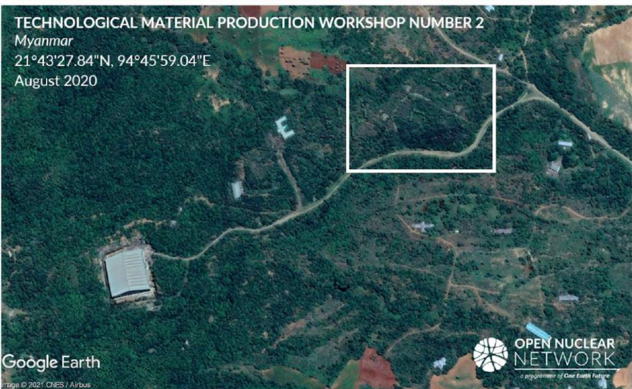
Figure 17. The Technological Material Production Workshop Number 2 appears to be left unattended, as evidenced most clearly by the three helipads (marked in white box) that have been slowly overgrown since 2010.
