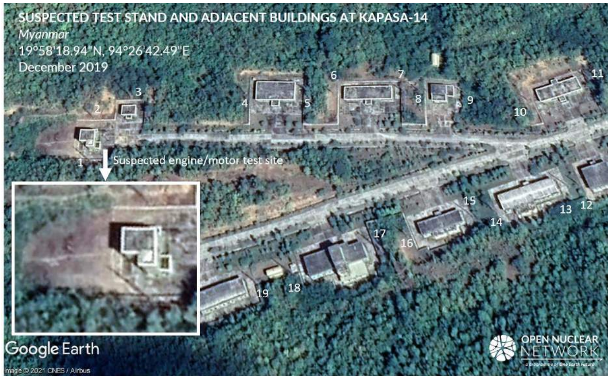
Figure 12. Multiple lightning rods (marked with numbers) are present at a building adjacent to a patch of barren land and nearby buildings. Image: Google Earth
